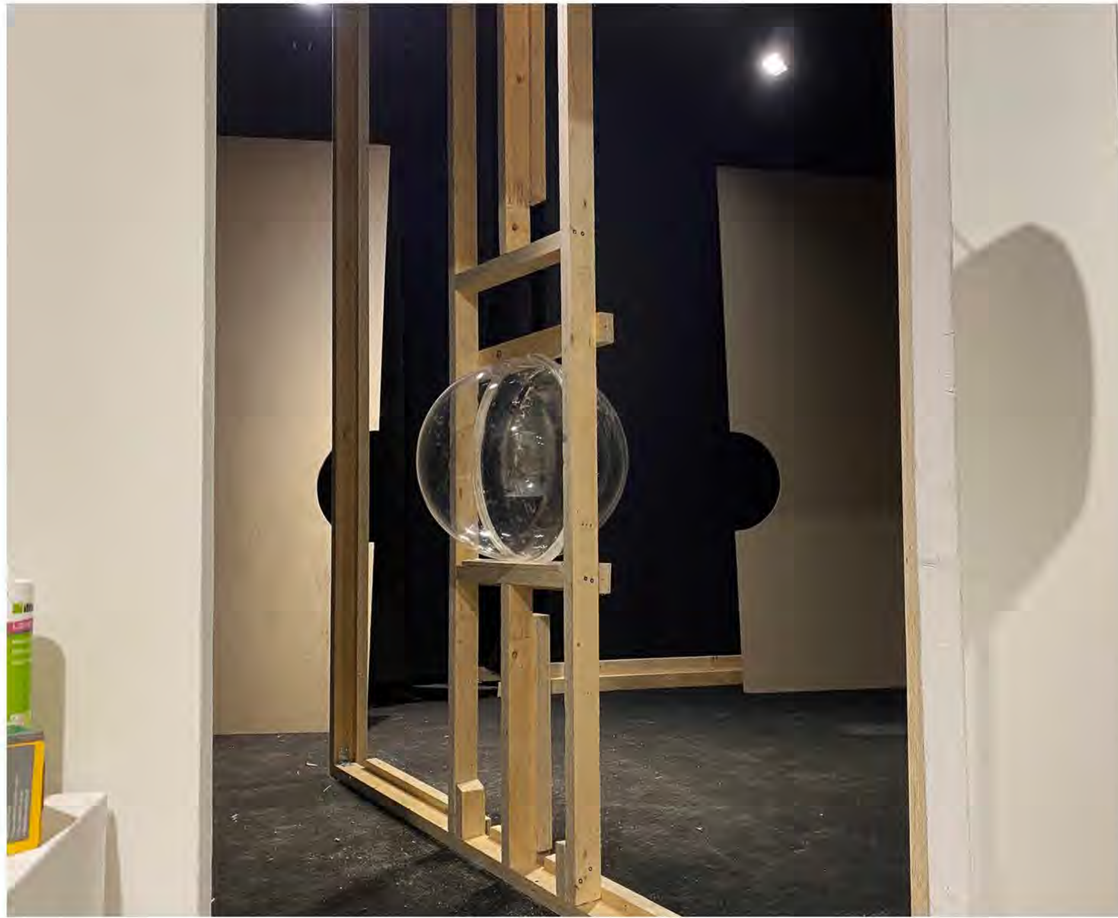
Photo documentation, process of construction: wall. Paola Fernanda Guzmán, May 2021
