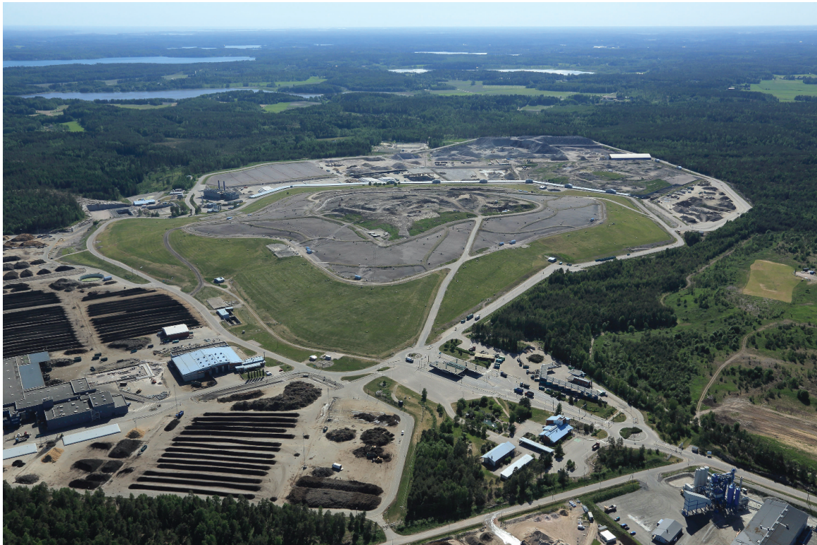
Figure 1. Ämmässuo waste treatment centre, a bird’s-eye view.
