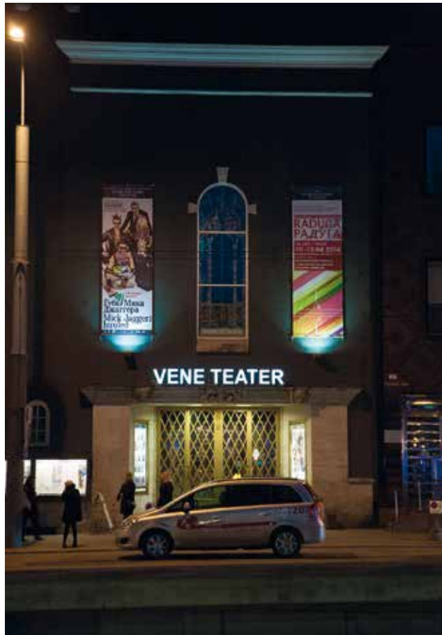
The facade on the Russian Theatre on the central square of Tallinn. Copyright Jelena Vilt.
