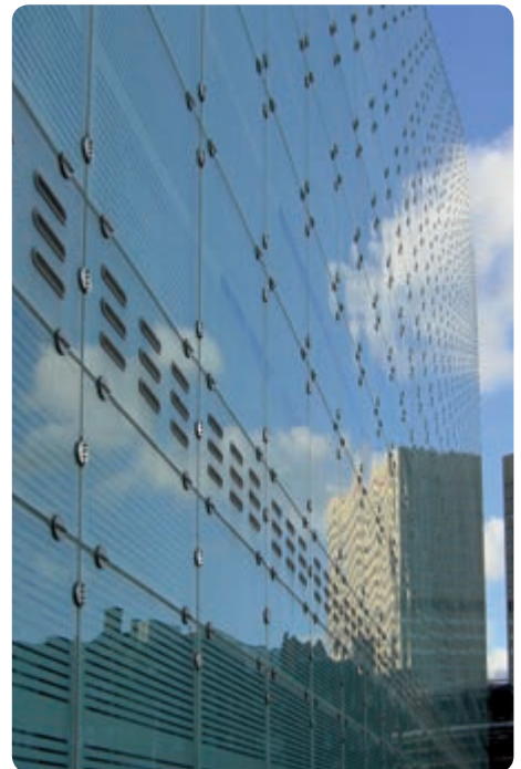
Ornamentation with constructional elements. Ian Simpson Architects. Urbis: The Museum of the Modern City, Manchester, 2002.
