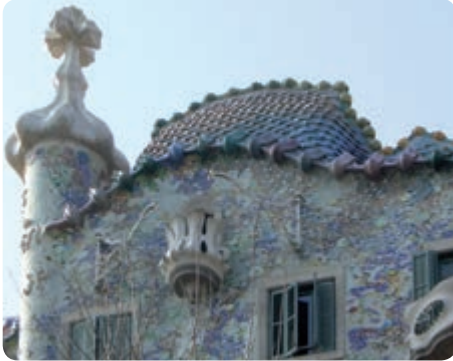
Ornamentation on the roof/ceiling. Antoni Gaudí: Casa Milà, Barcelona, 1910.
