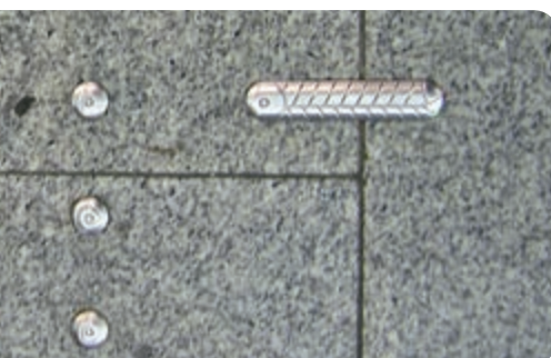
Ornament with a function. Walking map for the visually disabled on the floor of Kamppi bus station, Helsinki. Photographed in 2005.
