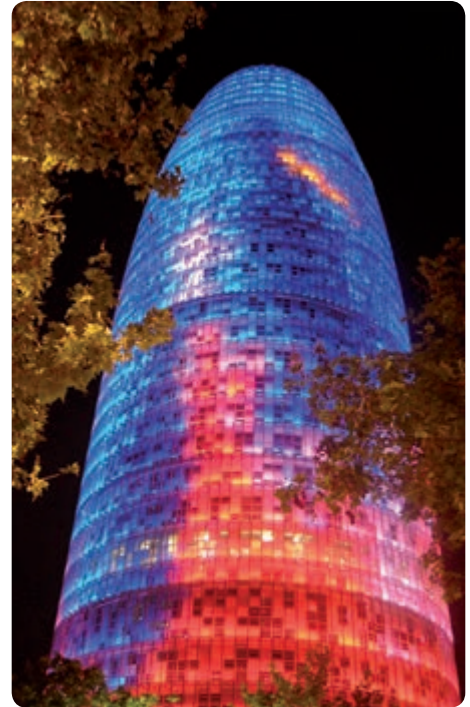
Mechanical structure as ornament. Jean Nouvel: Torre Agbar, Barcelona, 2005.
