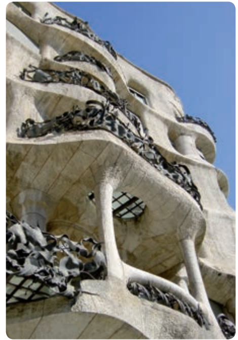
Antoni Gaudí: Casa Milà, Barcelona, 1910. The railings of the balconies, designed by Josep Maria Jujol, aim to give an impression of seaweed washed up onto the shore. Gaudí’s intention was that the residents would grow plants to enhance the visual effect.
